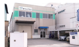
Moriguchi factory (Moriguchi-shi, Osaka, Japan)
