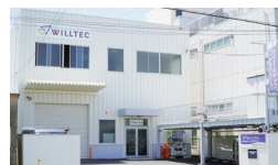
Moriguchi Factory (Moriguchi-shi, Osaka, Japan)
